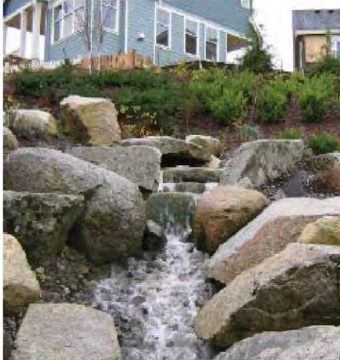
Figure 5.C.6-2. Example flow control system incorporated into the site design as an amenity, High Point West, Seattle
