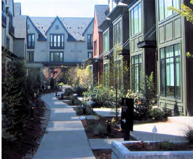
Figure 5.C.9.4. This residential complex incorporates passive surveillance, territorial definition, and good visibility and lighting to provide a more secure pathway and open space.
