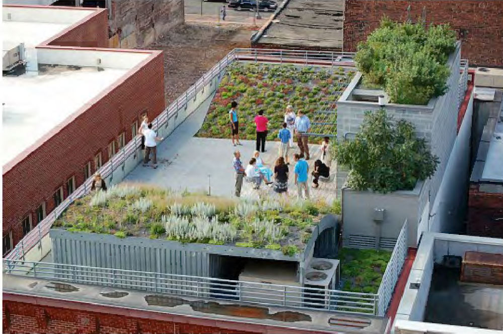
Figure 4.B.5.2-2. Green roofs can be used to hold and treat rainwater in ways that mimic natural systems.
