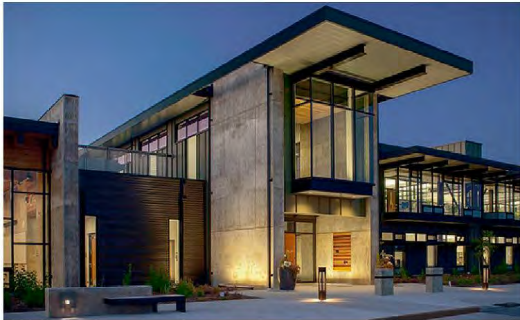
Figure 4.B.2.1-1. Good example of a clearly identified entrance and pedestrian access from the public street (image: AIA Southwest Washington).
