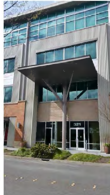
Figure 3.E.6.1-1. An industrial scaled entrance enhanced by details, lighting landscaping and materials.
