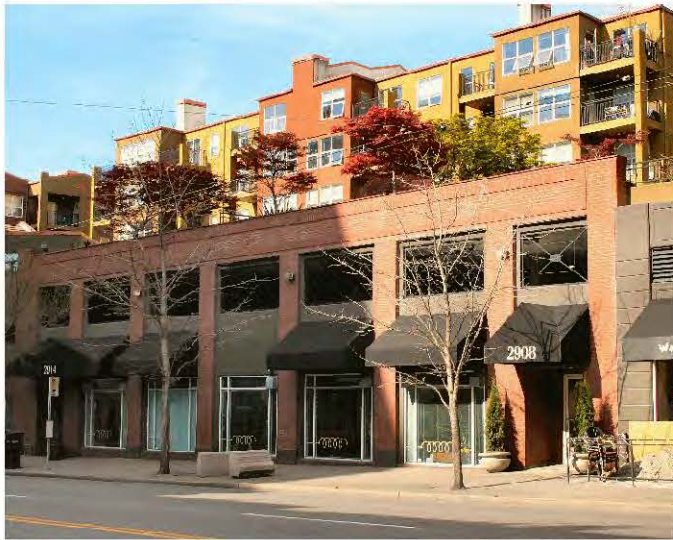
Figure 2.E.10.1-2. This building uses openings on its second level parking area to resemble windows.
