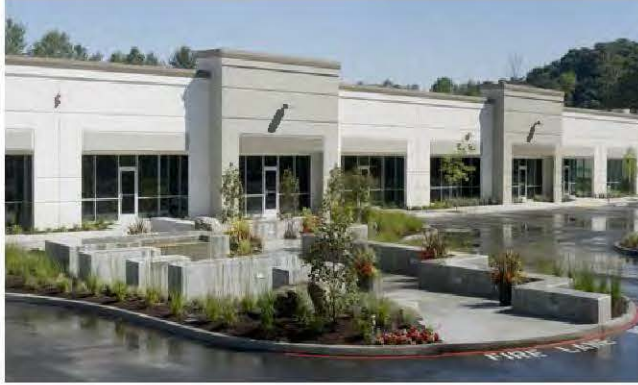
Figure 2.E.3.1-4. Industrial buildings can achieve an appropriate architectural scale through façade modulation and articulation, emphasis on the entrance, window patterns and landscaping.
