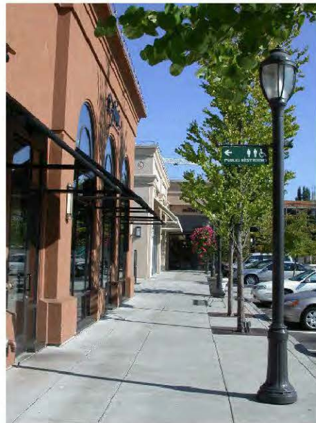
Figure 2.C.1.2-1. Example of a successful pedestrian sidewalk between parking lot and storefront.
