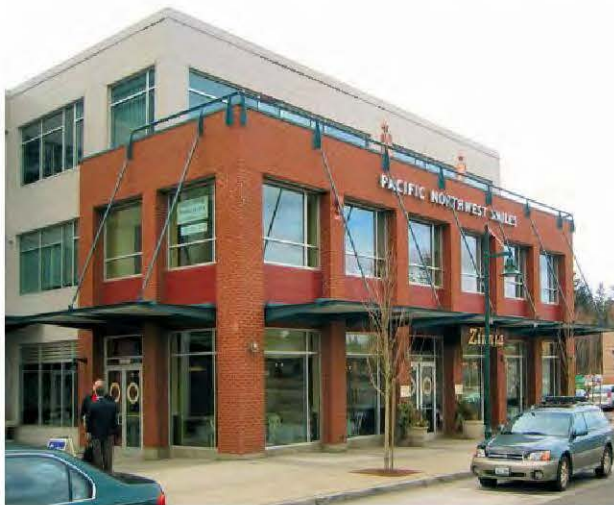
Figure 2.E.1.1-4. A successful application of approach 3: Contemporary forms and treatments. This example relates to its surroundings by using materials and colors compatible with adjacent buildings, breaking down the building's massing consistent with surrounding single story buildings, including a pedestrian street front to respond to its "main street" location, and fronting on wide, comfortable sidewalks.
