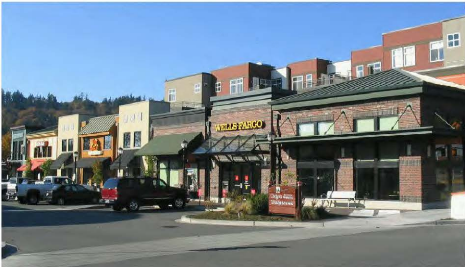
Figure 2.E.3.1-3. This development uses a variety of roof forms and heights and variations in roof textures by using metal hip roofs, different weather protection features, changing building materials and colors, and a modest amount of horizontal building modulation to reduce the overall architectural scale into smaller "storefront" components.
