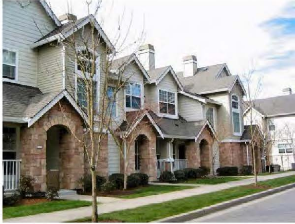
Figure 2.B.11.1-1. Desirable townhouse example. Units front on the street. Garages are off the alley.
