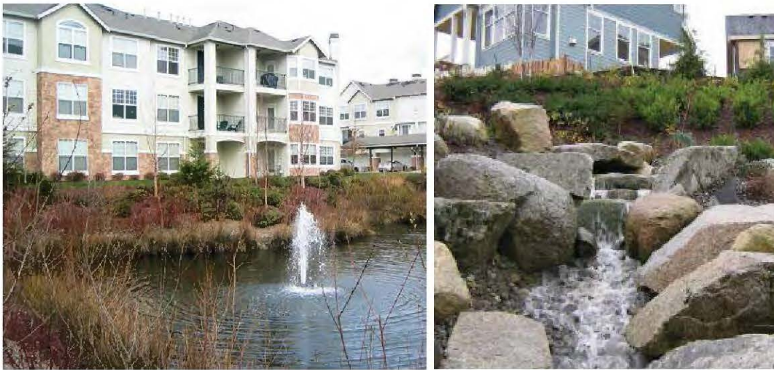
Figure 2.B.7.1-2: Example flow control system incorporated into the site design as an amenity, High Point West, Seattle
