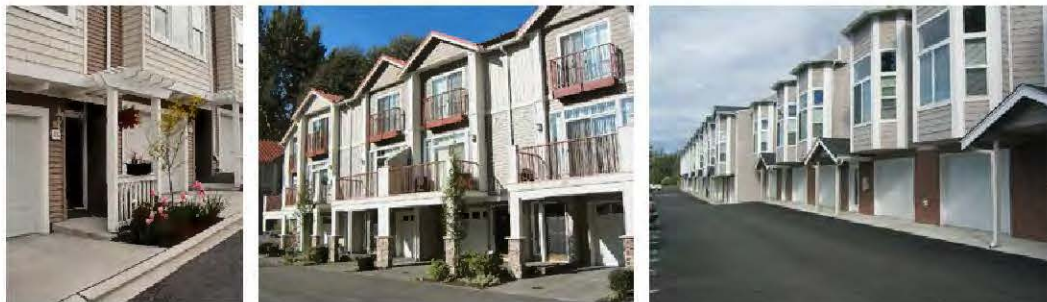
Figure 2.B.11.1-2. Good and bad examples of garage/entry configurations. The left example features a landscaped area and a trellis to highlight the entry. In the middle image, the balconies and landscaped areas de-emphasize the garage. In the bottom image, the lack of landscaping is a glaring omission.
