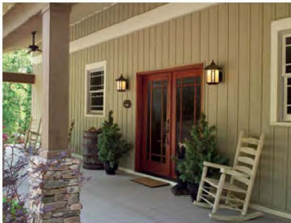
Figure 2.E.7.1-2. Fiber cement panels and similar materials are allowed when providing human scale details like this vertical siding.
