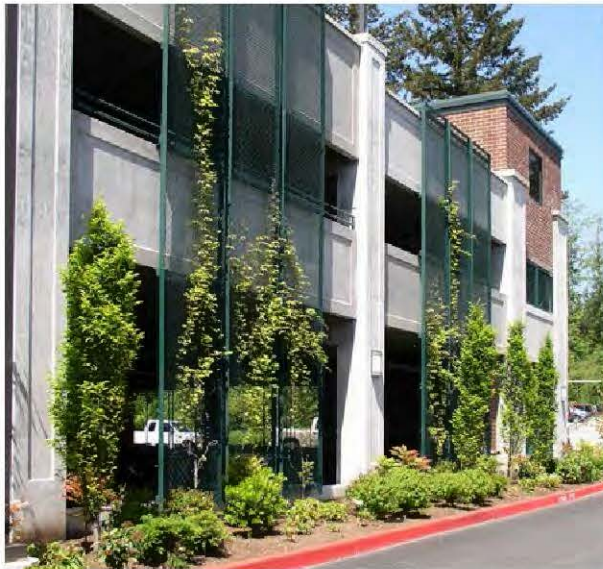
Figure 2.E.10.1-1. The side of this parking garage includes decorative grillwork, and a raised brick planter to enhance the pedestrian environment.
