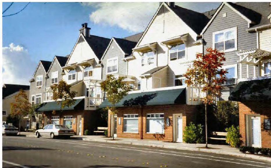
Figure 2.E.2.1-3 This mixed-use building incorporates decks, upper level setbacks, trellises, and landscaping to meet human scale guidelines.
