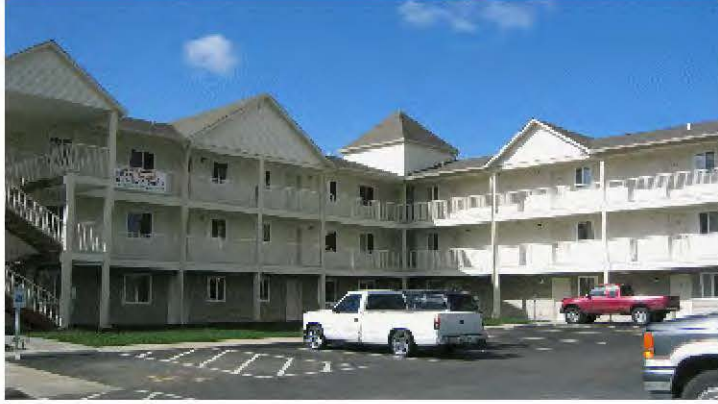
Figure 2.B.3.2-2. Elevated external walkways such as this are not allowed.
