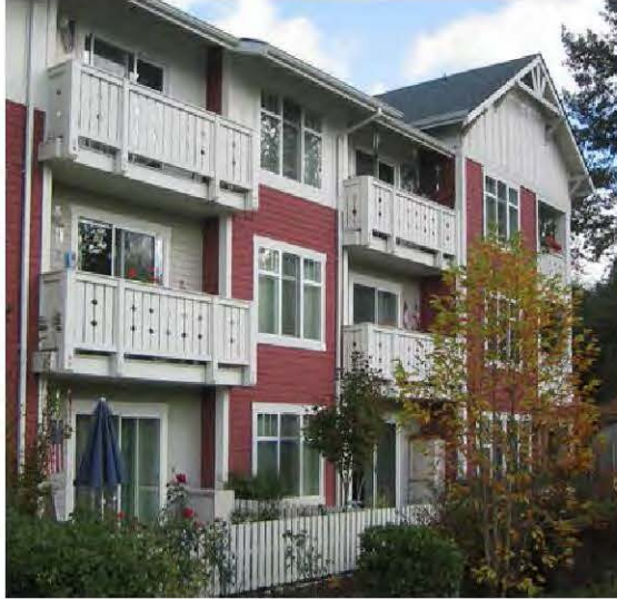
Figure 2.E.6.1-2. The multifamily building provides a number of details that enhance the pedestrian environment, including decorative railing, different siding treatments, window trim, balconies, eave detailing, lights, and opportunities for individual landscaping.
