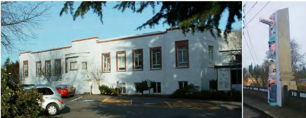
Figure 2.E.1.1-2. The DOT building on Capitol Boulevard and Tumwater Bridge Totems exemplify Art Deco architecture from the early to mid-1900s.
