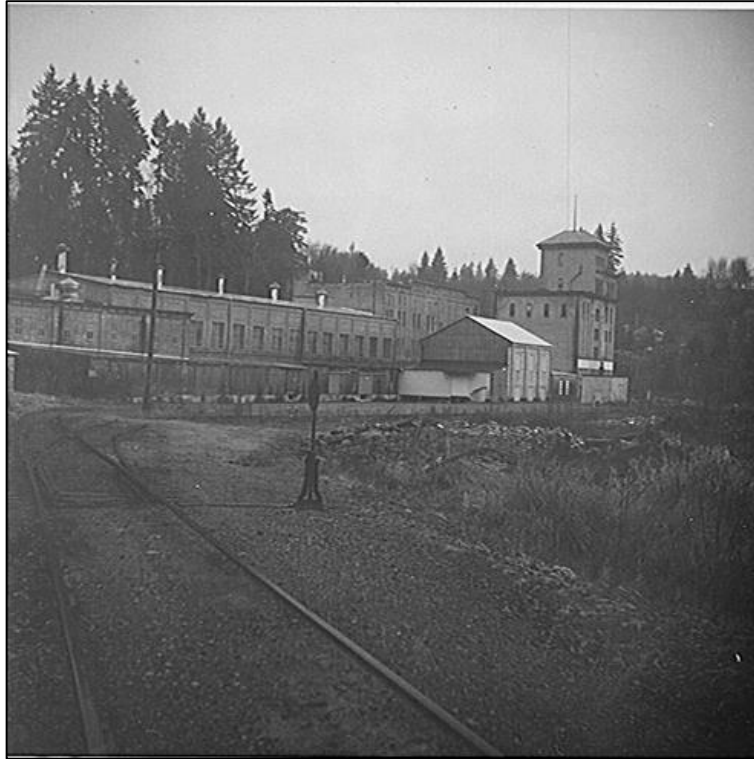
Figure 14. Old railroad spur is now a gravel road extending from the northeast corner of the Brewery complex along the hillside to the north, bisecting Wetland B.
