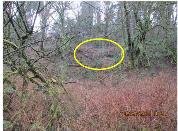
Figure B27. Slope failure on hillside by railroad.
