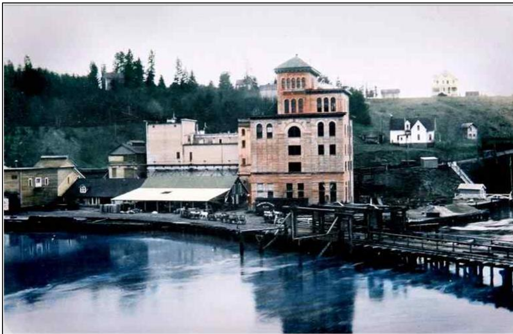
Figure 7. Photo from early 1900s showing bridge crossing the Deschutes River as well as other wooden structures associated with the Brewhouse complex.
