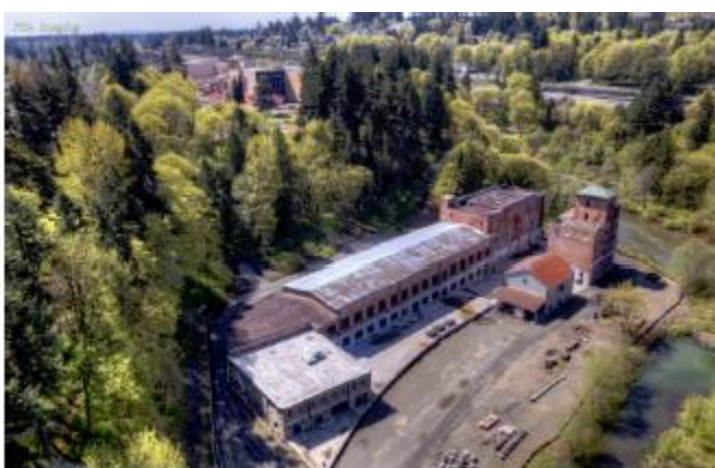
FIGURE 3.10-1 AERIAL VIEW OF BREWHOUSE
