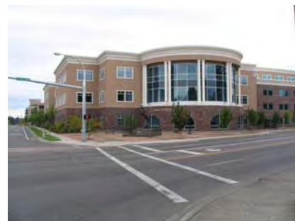
New office complexes, such as this one at the intersection of Capitol Blvd/Israel Rd, generate high peak hour traffic volumes, as well as creating need for pedestrian safety amenities.
