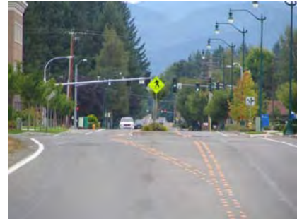
Israel Road SW - This urban collector connects minor and principal arterials, and provides access to Tumwater High School, a church, and local and state government facilities.
