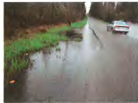
Water over the roadway at the sag in Kirsop Road
