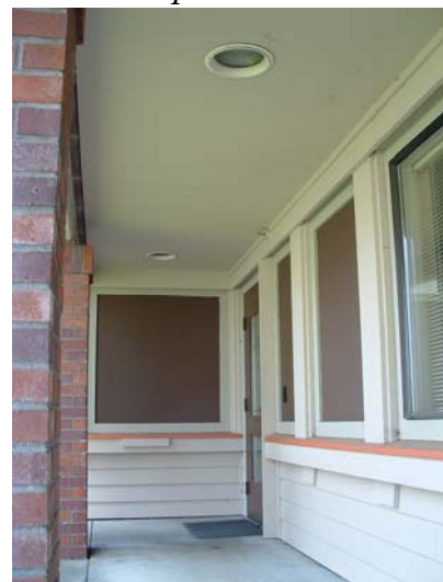
Fully shielded flush mount walkway lights at Tumwater City Hall
