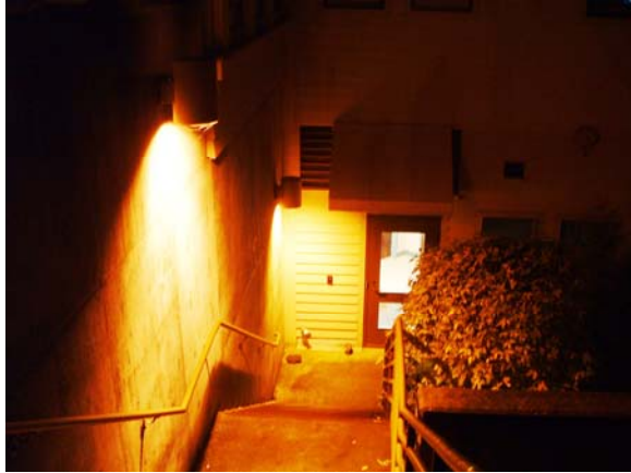
Low pressure sodium (City Hall steps)
