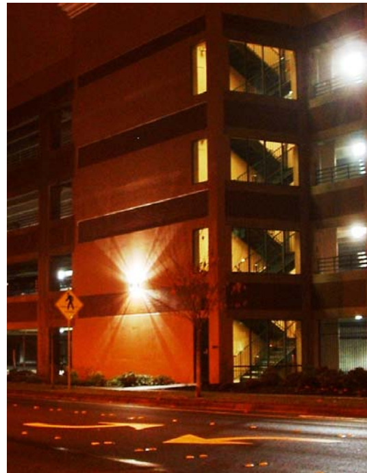
Wall box and parking garage lights Town Center East (Israel Road)
