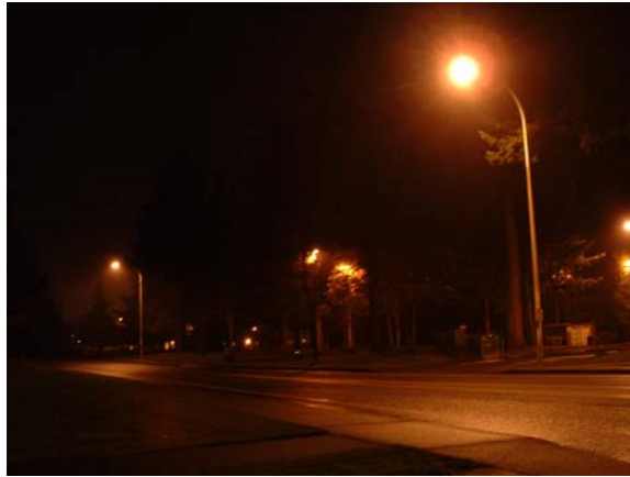
High pressure sodium (New Market Streetlights)
