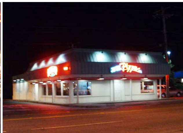
Downward fully shielded lighting Brewery City Pizza (Capitol Blvd)
