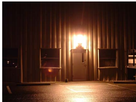
Bad: Tumwater Facilities Bldg (Israel Rd)
