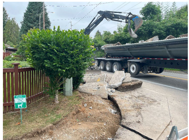
Sidewalk Demolition in Preparation for New Sidewalk Construction.
