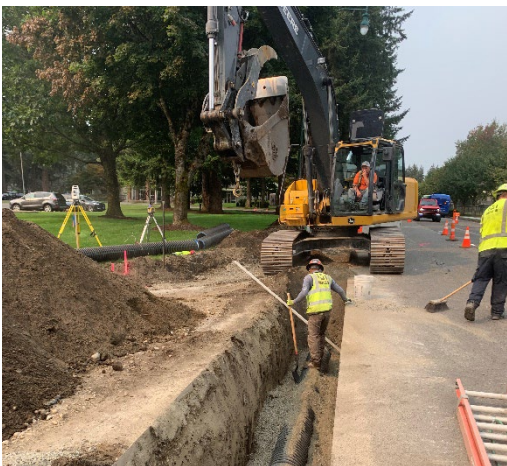
Israel Road Storm System Improvements
