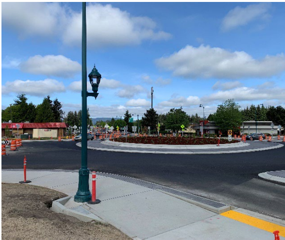
Capitol Boulevard and Trosper Road Roundabout – Looking Northwest
