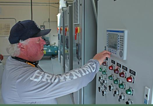
High-tech Supervisory Control and Data Acquisition (SCDA) equipment allows staff to continuously monitor the status of the production wells and the treatment system. The equipment is monitored 24 hours a day so adjustments can be made promptly if needed.
