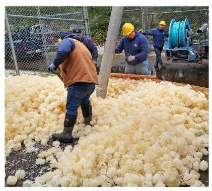
Your water quality crews have a lot of fun at their work! These aeration balls at towers located at the Bush and Palermo wellfields must be replaced every 10 years. In 2023, over 123,000 balls were replaced at the Bush tower.
