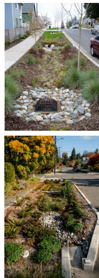
Bioretention Examples (Seattle, Washington)
