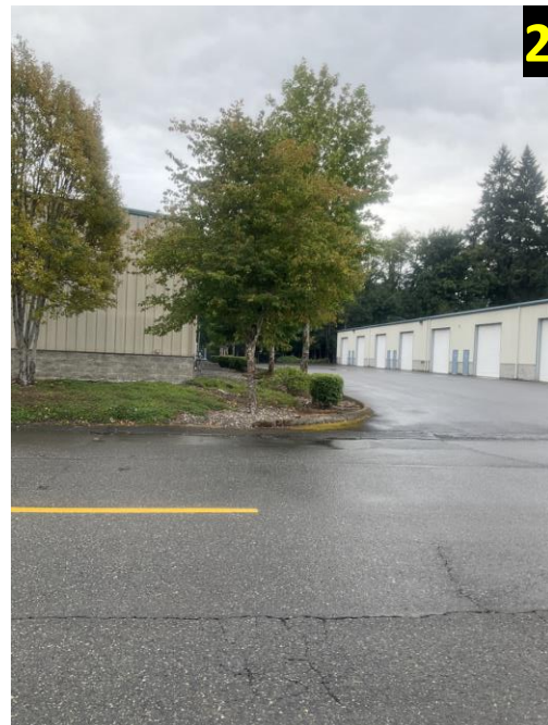
Facing South (South of 37th Ave SW)
