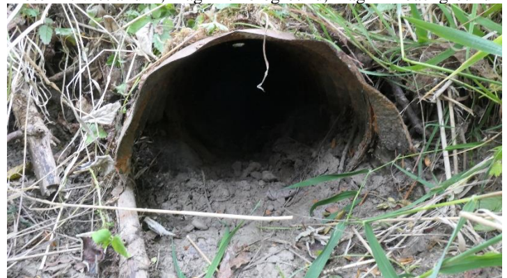
Photo 16. Culvert between Wetlands A & B
