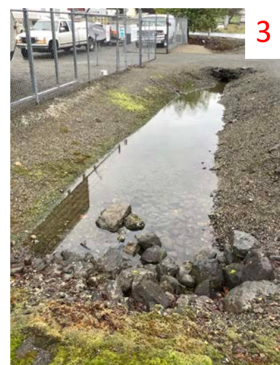
Gravel-lined Ditch on Lambskin Facing North
