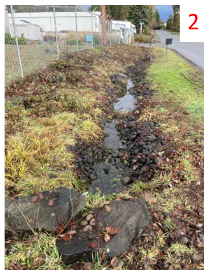
2 Gravel-lined Ditch between Troser and 51st Facing North
