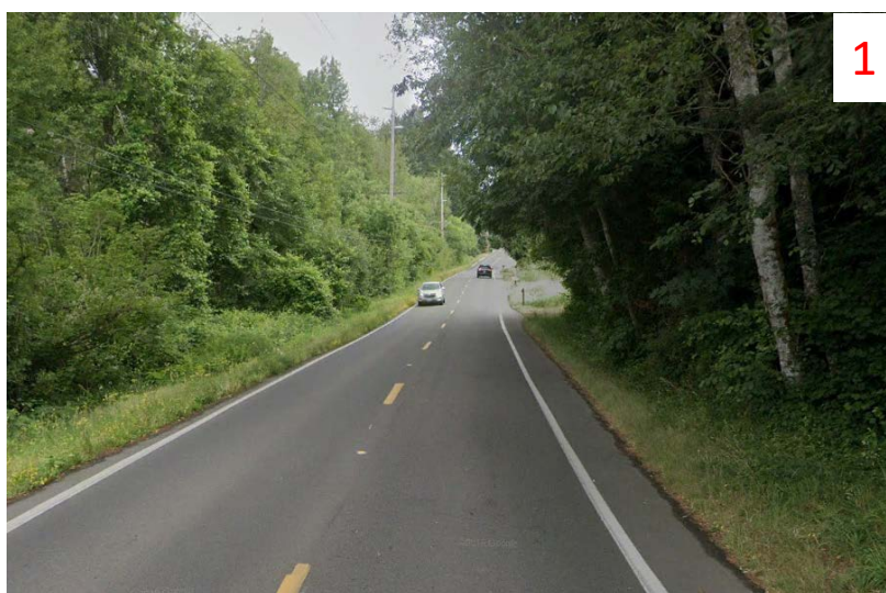
5316 Rural Road SW Facing North (Photo Courtesy of Google Earth)
