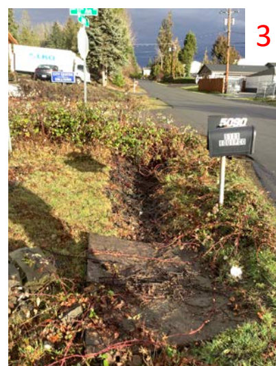
3 Small Ditch on the Corner of 51st and Joppa Facing North
