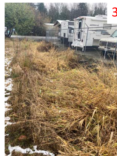
Tire-lined Ditch Facing West
