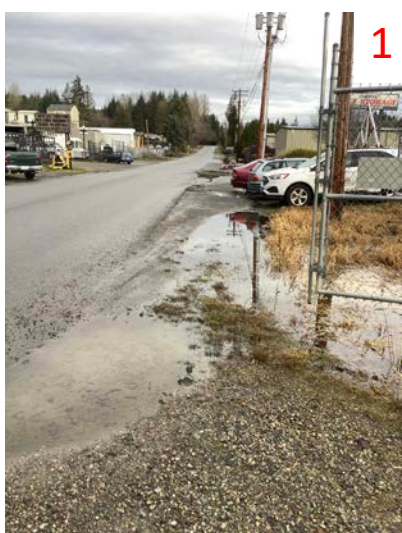
Ponding on the Southeast Corner of Troser and Joppa Facing North
