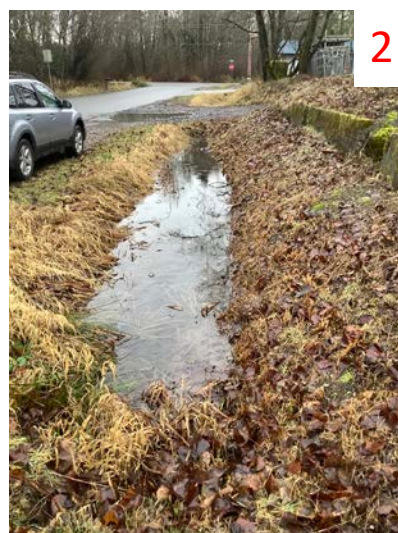
Grass-lined Ditch on Lambskin Facing South
