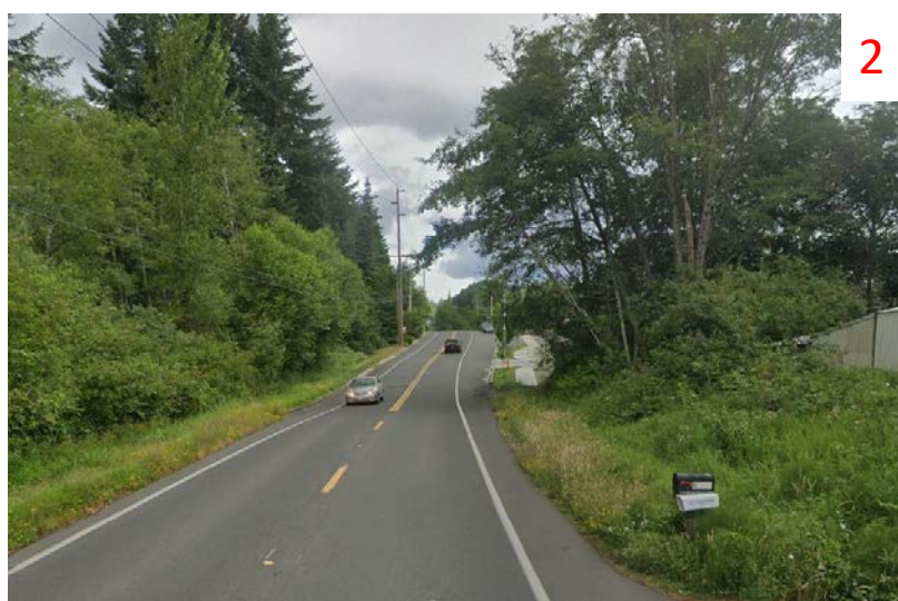
4856 Rural Road SW Facing North (Photo Courtesy of Google Earth)
