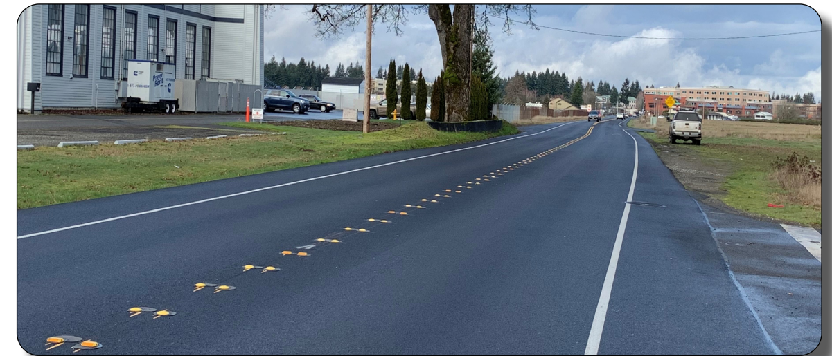
Resurfacing Old Hwy 99 Looking North (2019)
