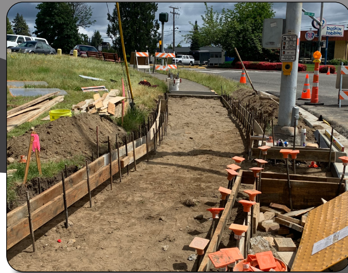
New Sidewalk and Curb – Capitol Blvd and Custer Way (2020)
