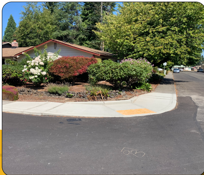
New ADA-Compliant Pedestrian Curb Ramp (2021)
