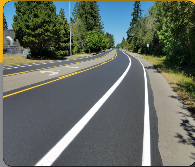
RW Johnson Blvd, Completed Mill and Inlay (2018)
