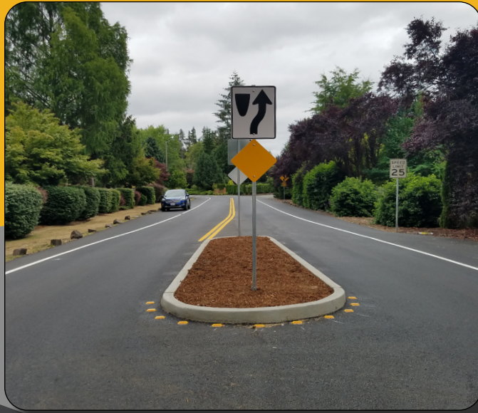
Completed Median on Miner Drive (2018)
