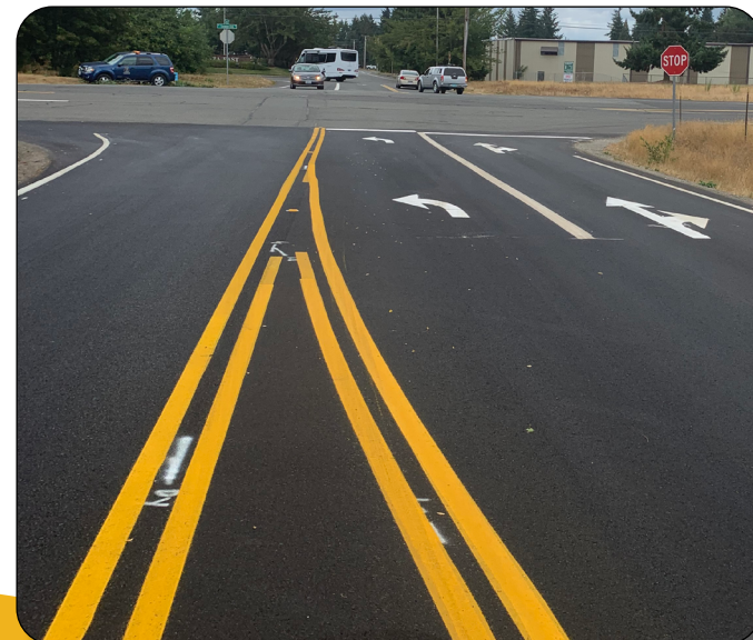
Pavement Markings at Bonniewood and Tumwater Blvd (2021)
