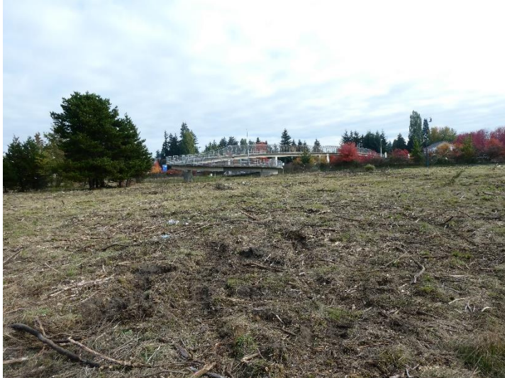
Photo 3. Pedestrian structure bordering the subject property
