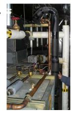
economizer and second-stage cooling for this and all the other air handlers in the building is provided by ground-mounted direct-expansion (DX) condensing units. Heating is provided by a hot water coil supplied by the boilers for all air handlers. The main unit serving the first floor runs 24/7 in order to condition the police station, which is occupied 24/7.
