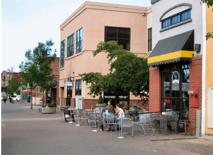
Figure E.9.2-1. Example of secondary public access. Note the planters, window sign, and awning.
