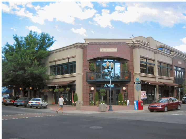
Figure E.5.1-1. To emphasize its street corner location, this building uses a cropped corner, change in building materials, decorative façade elements, and a modulated roofline.
