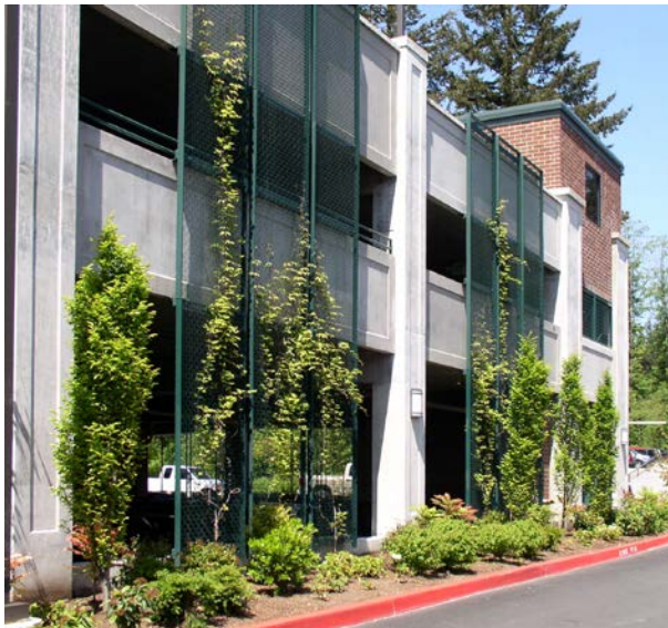
Figure E.10.1-1. The side of this parking garage includes some decorative grillwork and a raised brick planter to enhance the pedestrian environment.
