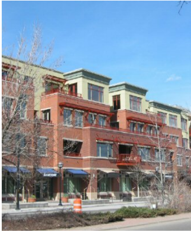
Figure E.3-2. Example of a well articulated building. Note how the awnings, window divisions, pilasters columns and cornice line all serve to divide up the façade into smaller segments without disrupting the unity of the overall design.
