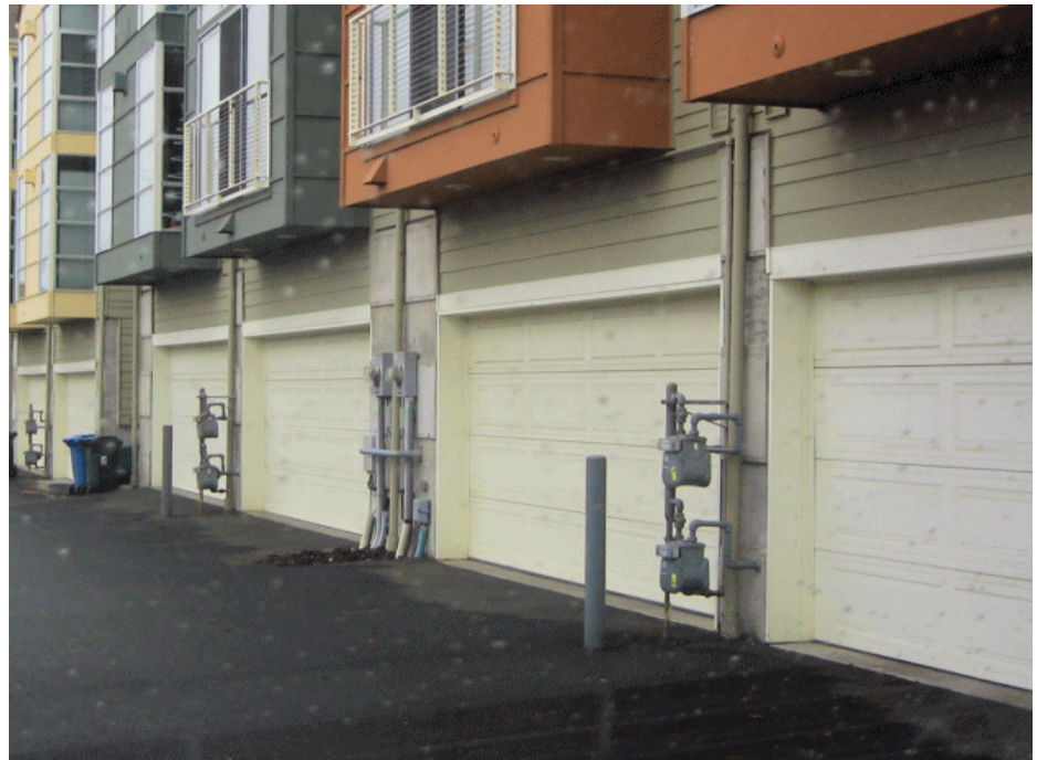
Figure B.5.1-3. Place utility meters in less visible locations. Note that this example is acceptable on a service alley but not near a street or residential walkway.
