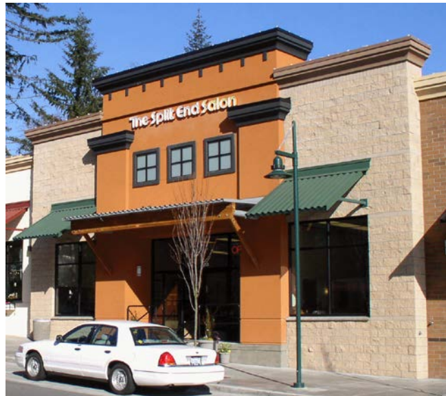
Figure E.7.1-1. This storefront effectively combines EIFS and concrete block with wood trim and metal detailing.
