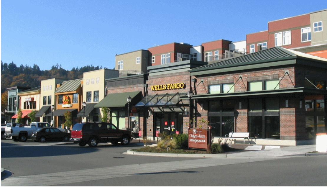
Figure E.3-3. This development uses a variety of roof forms and heights and variations in roof textures by using metal hip roofs, different weather protection features, changing building materials and colors, and a modest amount of horizontal building modulation to reduce the overall architectural scale into smaller “storefront” components.
