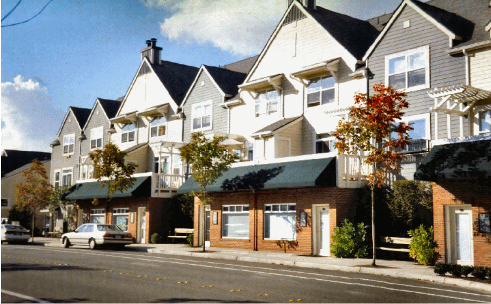
Figure.E.2.1-3 This mixed-use building incorporates decks, upper level setbacks, trellises, and landscaping to meet human scale guidelines.
