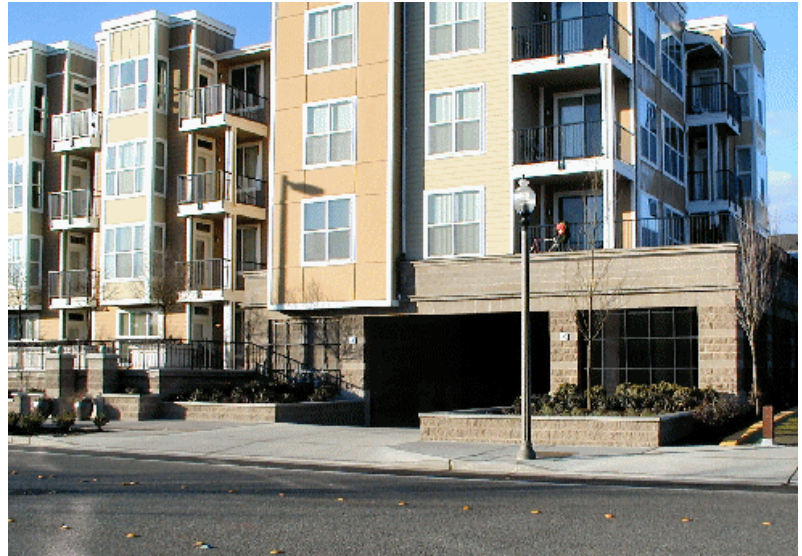
Figure E.10.1-3. Design parking garages to obscure the view of parked cars. Note the landscaping that separates the garage from pedestrians.
