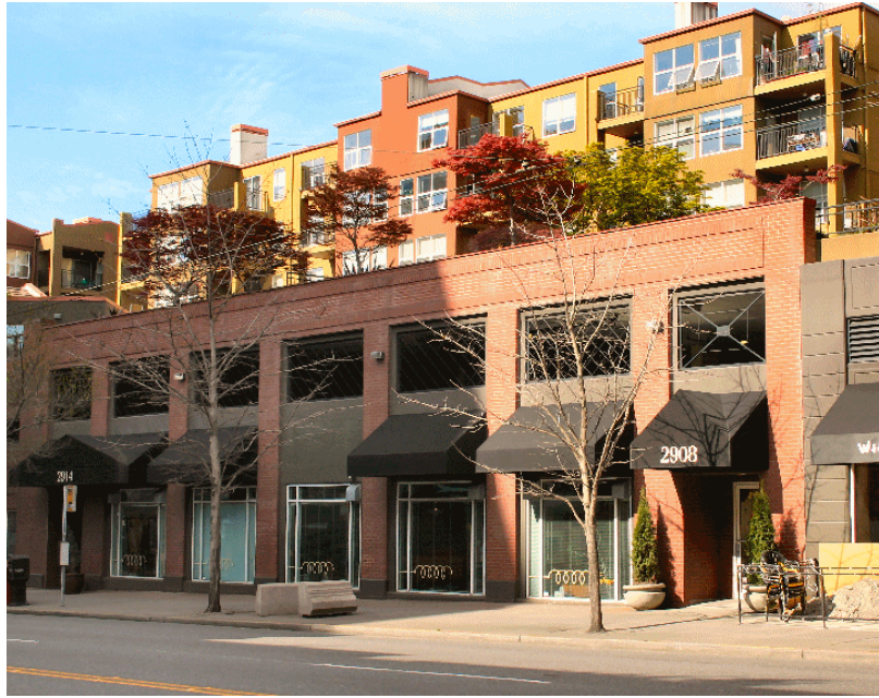
Figure E.10.1-2. This building uses openings on its second level parking area to resemble windows.
