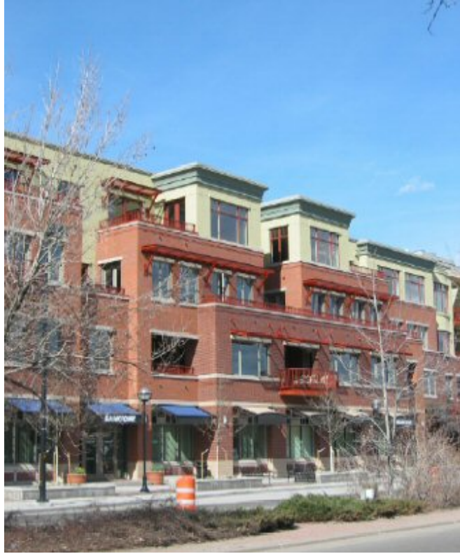
Figure E.3.1-1. Mixed-use building with modulation to increase its interest and human scale.
