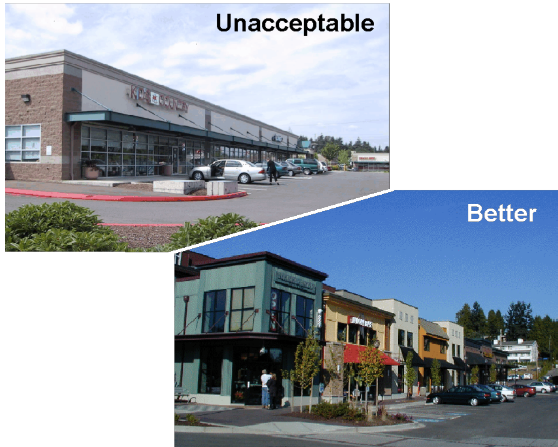
Figure E.4.2-3. The continuous canopy on top is monotonous and deemphasizes individual storefronts. The bottom example provides a variety of weather protection features and represents a more desirable example.
