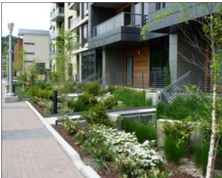
Figure B.6.1-1 A preferred method of handling storm water is through retention systems, such as rain gardens, incorporated as site amenities. Other low-impact development techniques are encouraged, and in many cases, required.
