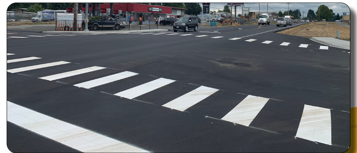
Intersection of Old Highway 99 and Henderson Boulevard
