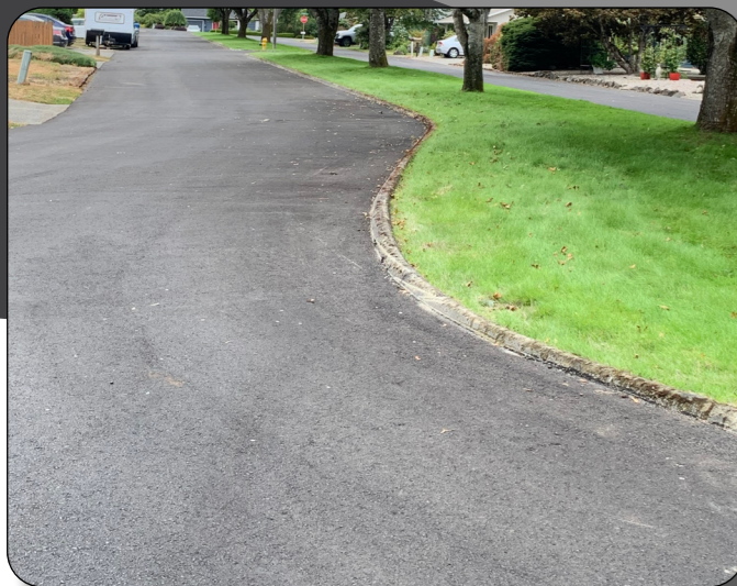
New asphalt pavement on Maplewood Lane
