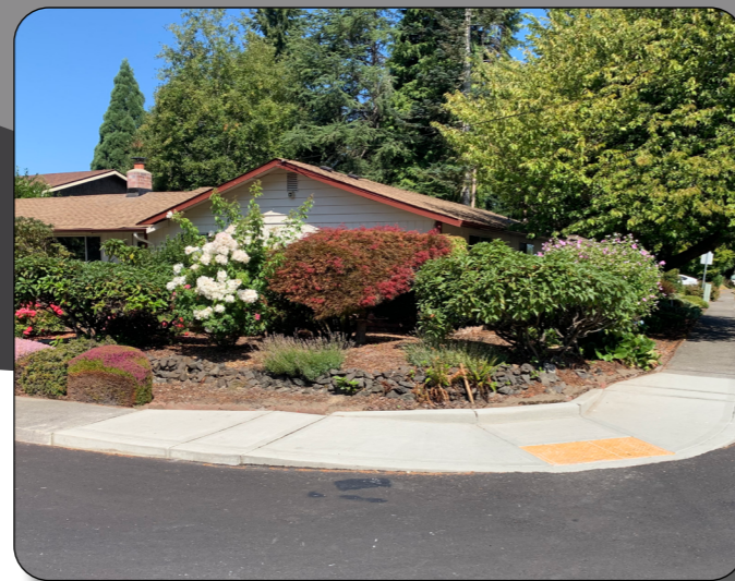
New ADA-compliant pedestrian curb ramp
