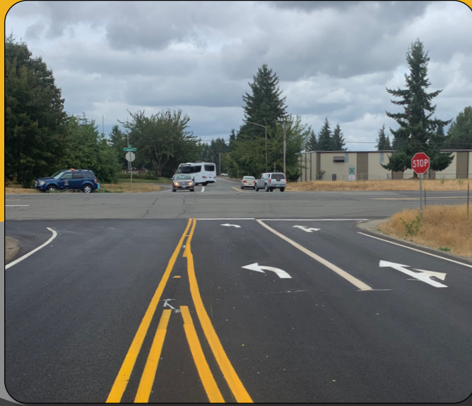
Pavement markings at Bonniewood and Tumwater Blvd
