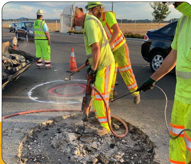
Adjustment of a valve box
