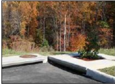
1. Inspection of Filterra and surrounding area
