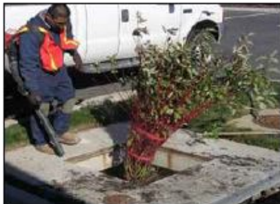
5. Clean area around Filterra
