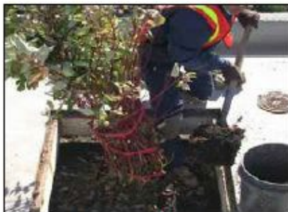
3. Removal of debris, trash and mulch
