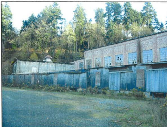
North Facade of Brewhouse Complex
