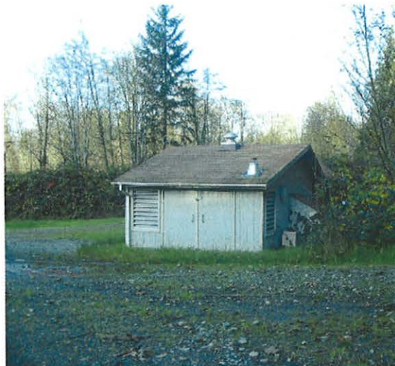
Sewer Lift Station
