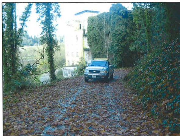
Boston Street Approaching Brewhouse
