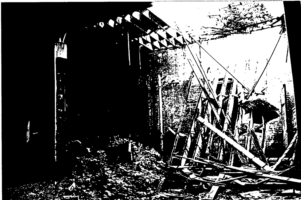
Collapsed roof in Brewhouse building
