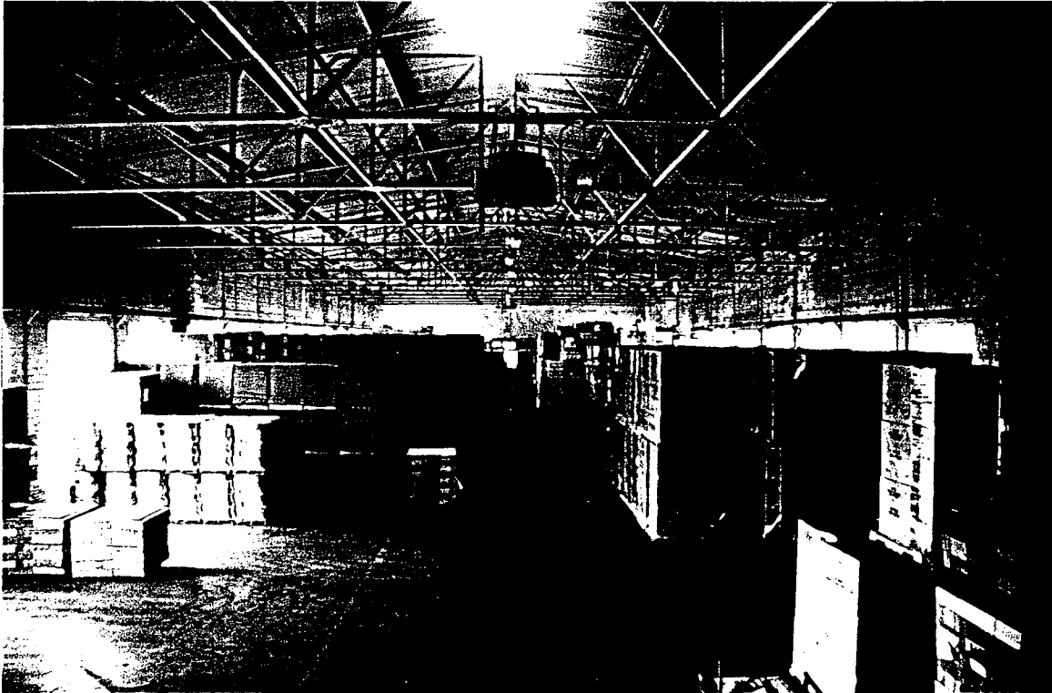
Second floor warehouse area of East Addition Warehouse
