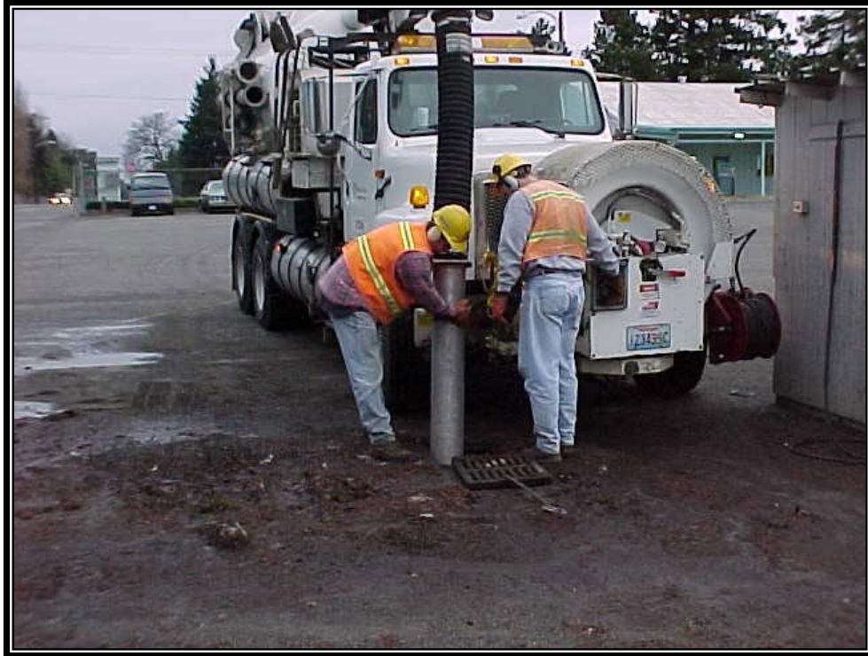
Figure 4.23. Catch Basin Cleaning with a Vacuum Truck.
