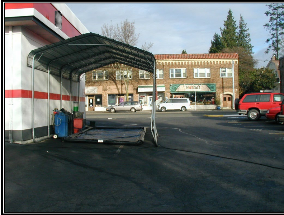
(Photo courtesy of Seattle Public Utilities)
