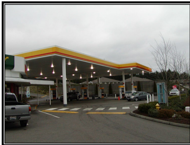
Figure 5.3. Roof at Fueling Island To Prevent Stormwater Run-On.
