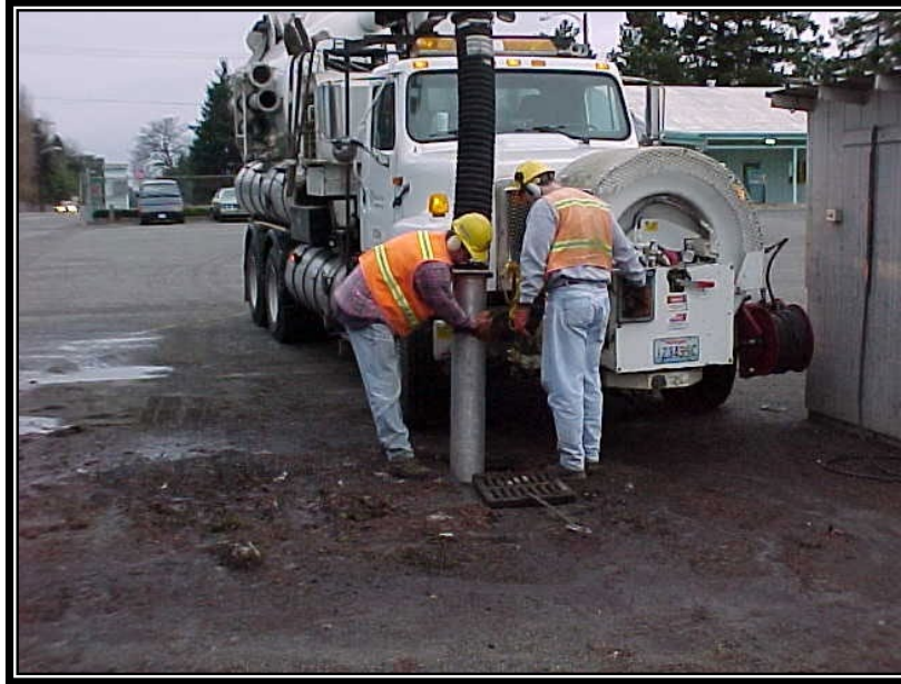
Figure 5.8. Catch Basin Cleaning with a Vacuum Truck.
