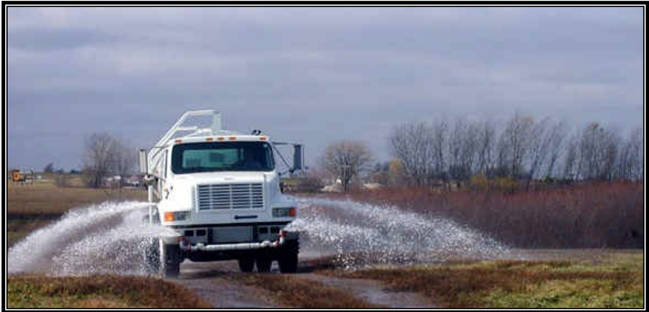
Figure 4.21. Dust Suppression by Water Spray.
