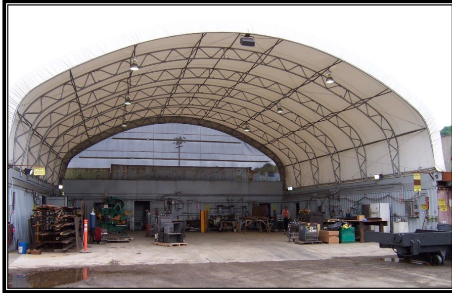
(Photo courtesy of Seattle Public Utilities)
