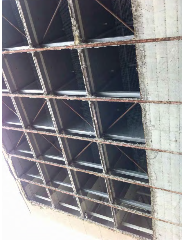
T Cellar with exterior removed
