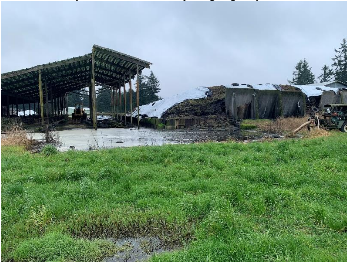
Photo 3. Agricultural buildings onsite
