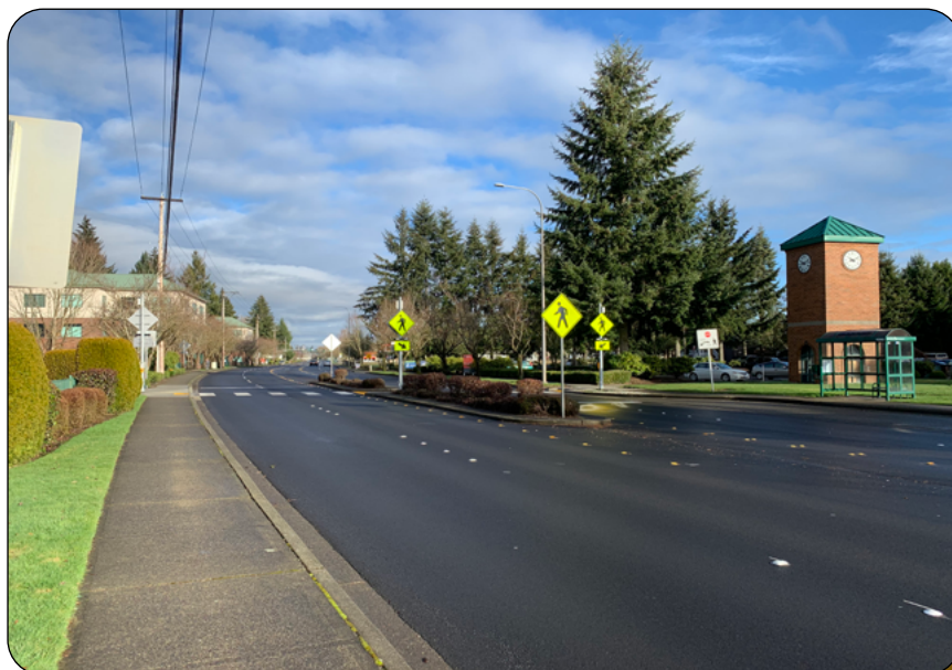
Finished crosswalk on Capitol Boulevard
