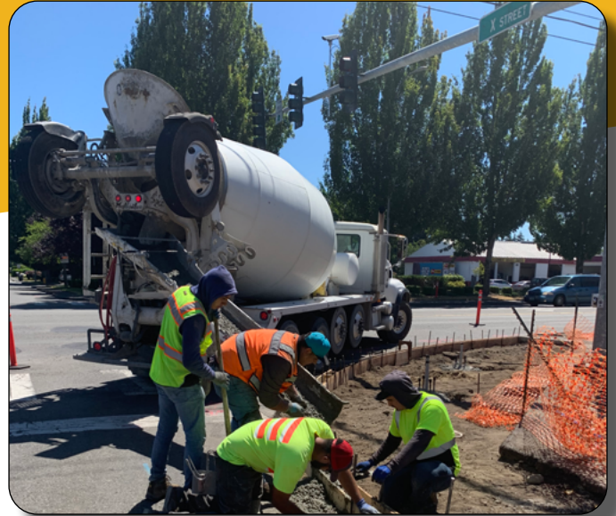
Pouring new curb—Capitol Blvd and X Street
