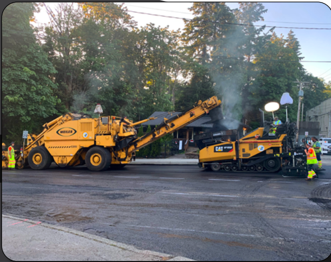
Paving machines working at Custer Way
