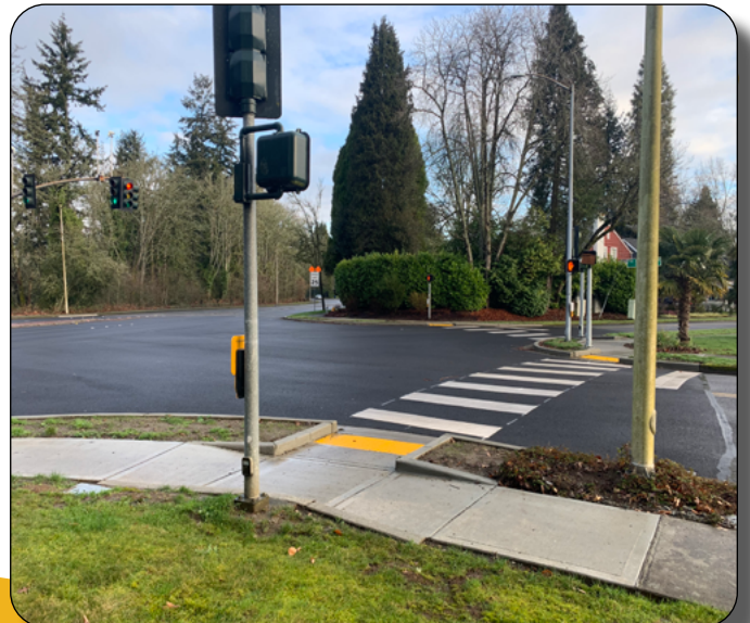
Finished crosswalks—Capitol Blvd and Carlyon Ave/Sunset Way
