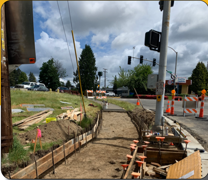
New sidewalk and curb—Capitol Blvd and Custer Way
