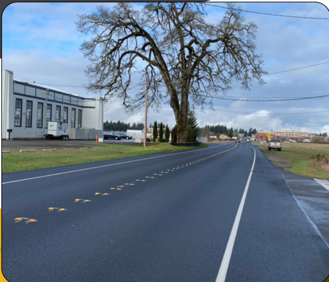
Finished project – Old Highway 99
