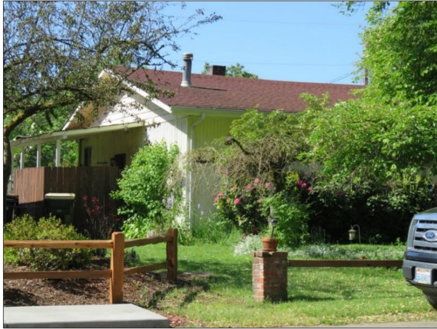
Figure 7-27. 113 Linda St. SE, north and east elevations; view southwest.
