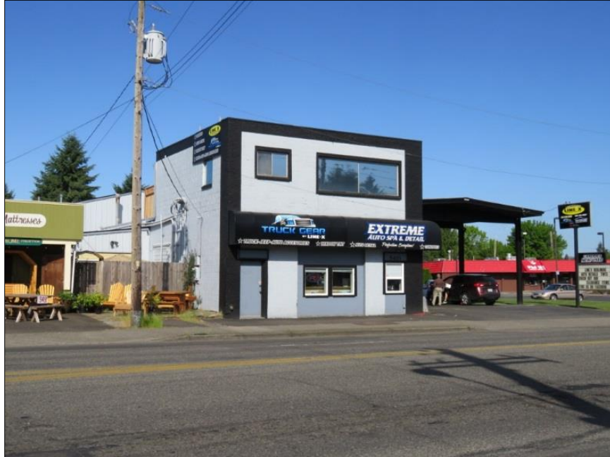
Figure 7-23. 5403 Capitol Blvd. SE, south and east elevations; view northwest.
