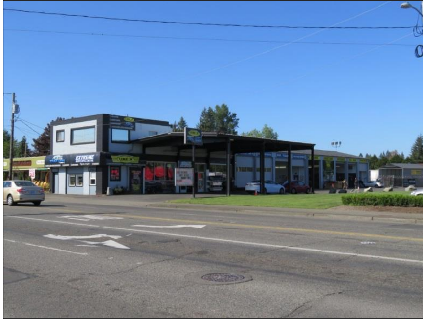
Figure 7-22. 5403 Capitol Blvd. SE, north elevation; view southwest.
