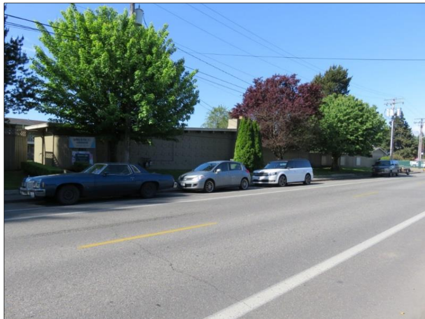
Figure 7-9. The north-facing façade of the office building at 301 Lee St. SW; view southwest.
