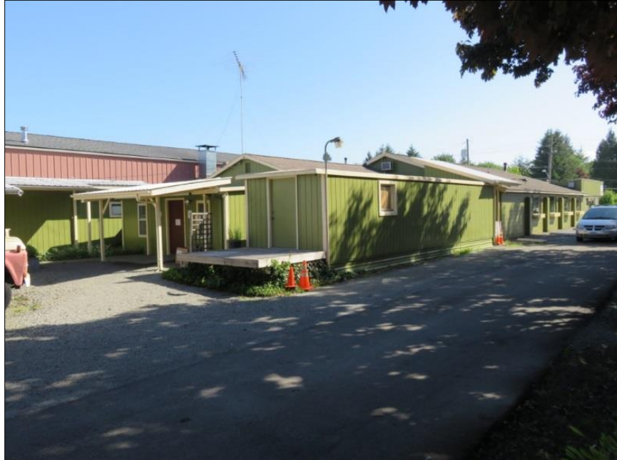
Figure 7-19. 5407 Capitol Blvd. SE, rear ( west ) elevation; view northeast.
