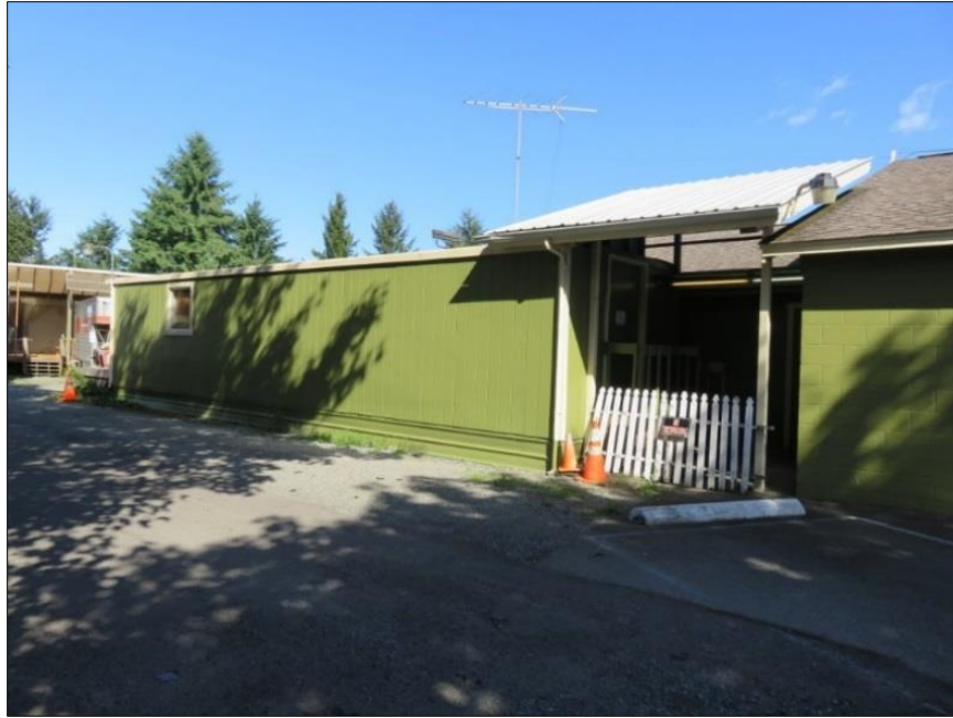
Figure 7-18. 5407 Capitol Blvd. SE, south elevation; view northwest.
