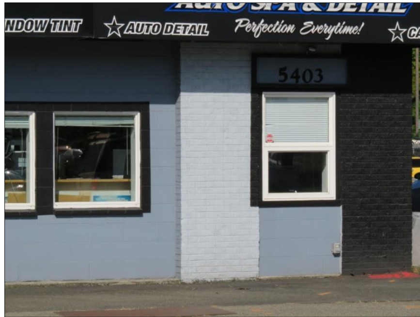
Figure 7-24. 5403 Capitol Blvd. SE, façade detail; view west.
