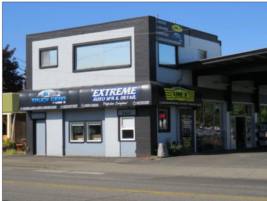
Figure 7-21. 5403 Capitol Blvd. SE, east and north elevations; view southwest.
