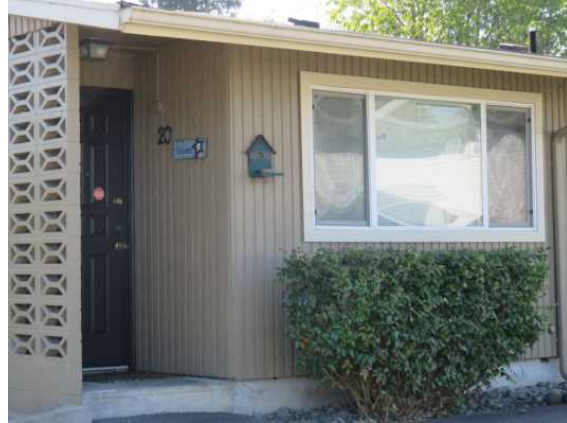
Entry details at 301 Lee St. SW
