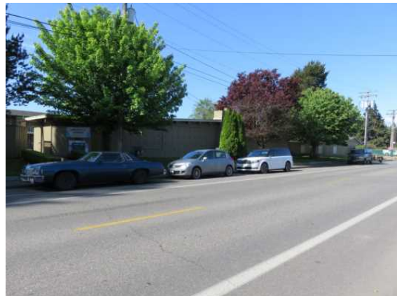
North-face of the office building at 301 Lee St. SW
