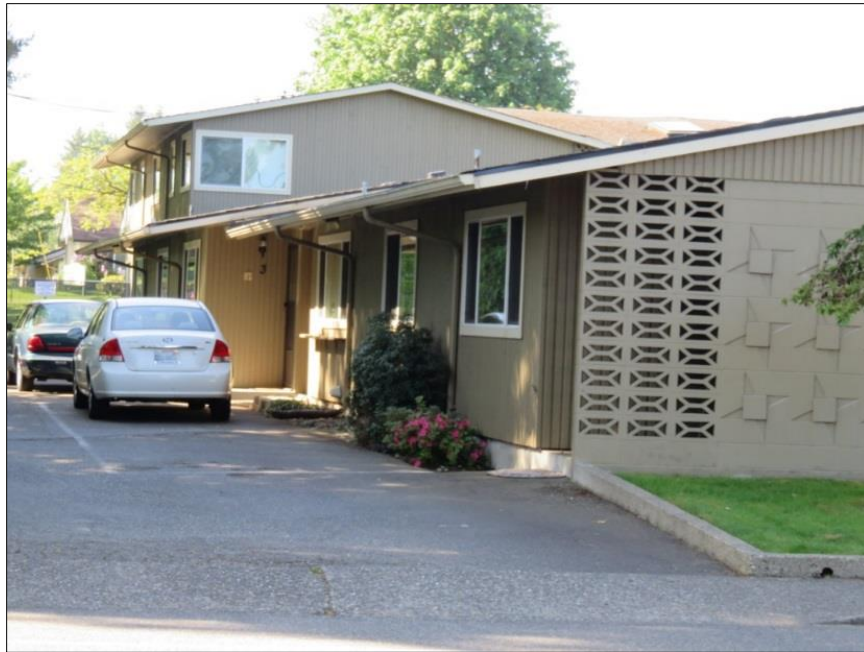
Figure 7-12. 301 Lee St. SW, single-story and two-story apartments along the east wall of the complex; view southwest.
