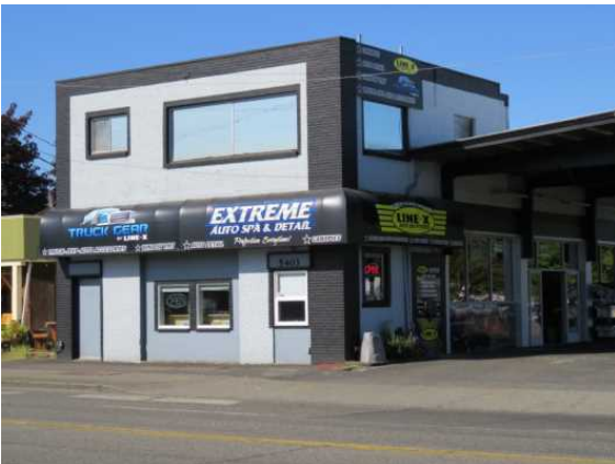
5403 Capitol Blvd. SE, east and north elevations
