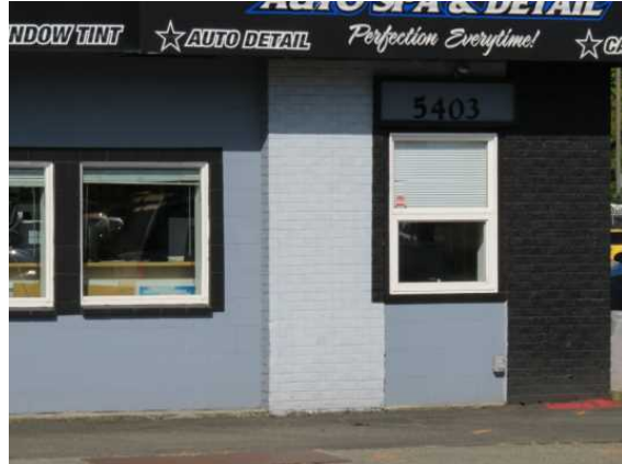
5403 Capitol Blvd. SE, façade detail
