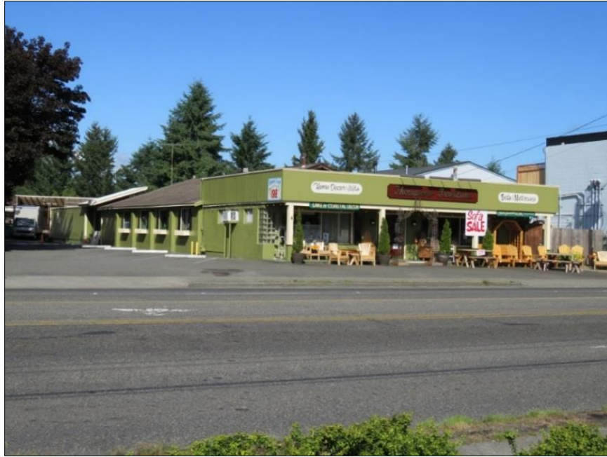
Figure 7-14. 5407 Capitol Blvd. SE, façade and south elevation; view northeast.
