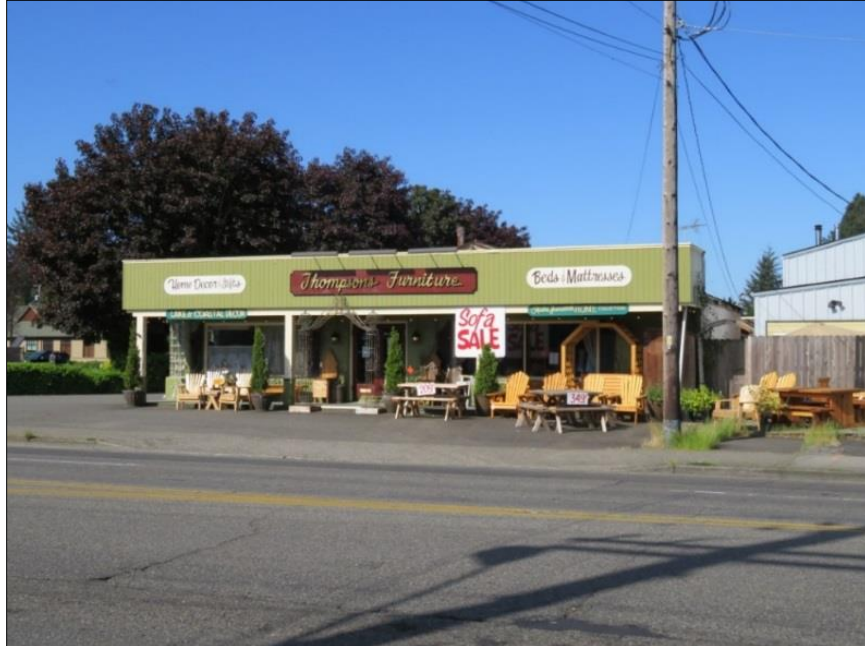
Figure 7-15. 5407 Capitol Blvd. SE, façade; view west.
