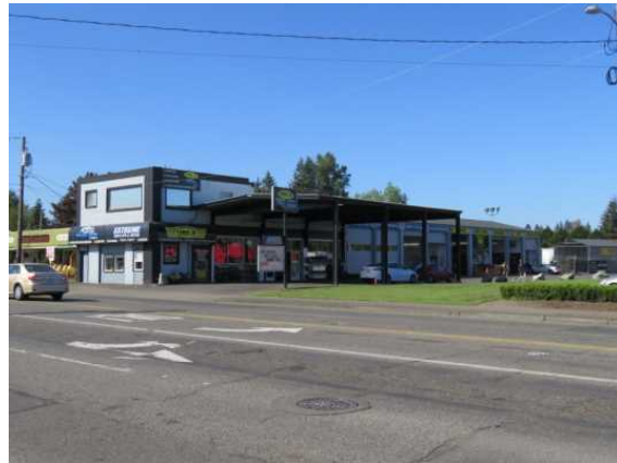
5403 Capitol Blvd. SE, north elevation
