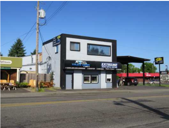
5403 Capitol Blvd. SE, south and east elevations
