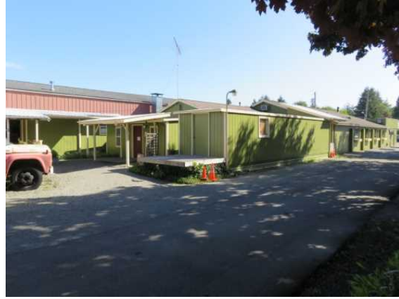
5407 Capitol Blvd. SE, rear (west) elevation
