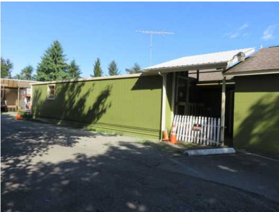
5407 Capitol Blvd. SE, south elevation
