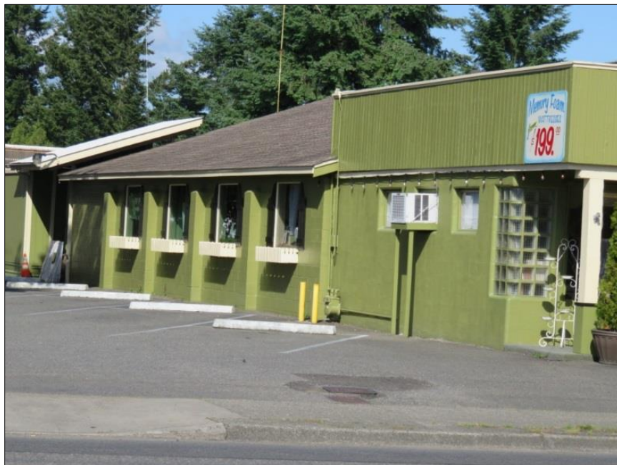
Figure 7-17. 5407 Capitol Blvd. SE, south elevation; view northwest.
