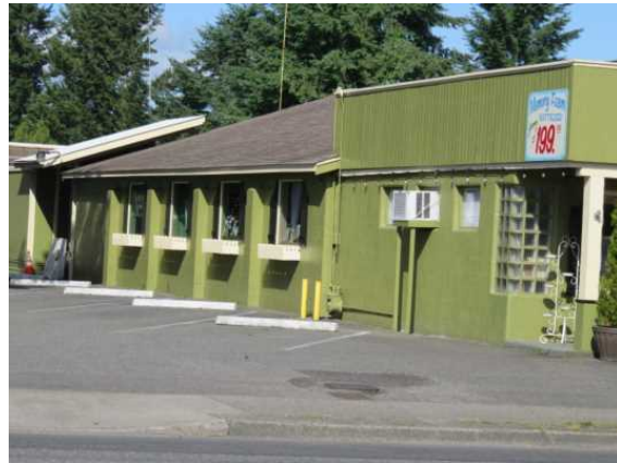
5407 Capitol Blvd. SE, south elevation
