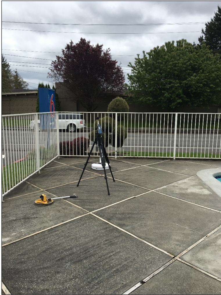
3. V-2, Motel 6 pool area facing south toward Lee Street.
