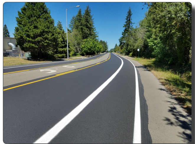
RW Johnson Blvd, Completed Mill and Inlay
