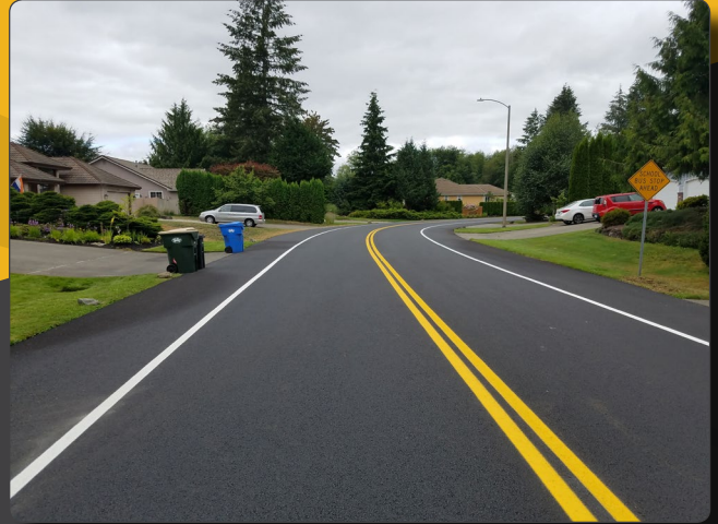
Completed Overlay on Miner Drive
