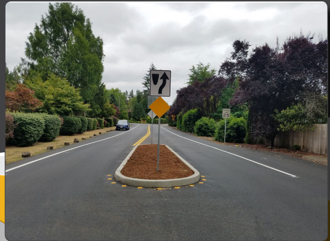
Completed Median on Miner Drive
