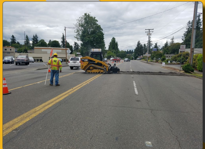
Capitol Boulevard Joint Grinding
