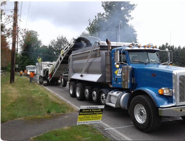
70th Ave at Kirsop Rd, Planing Existing Asphalt
