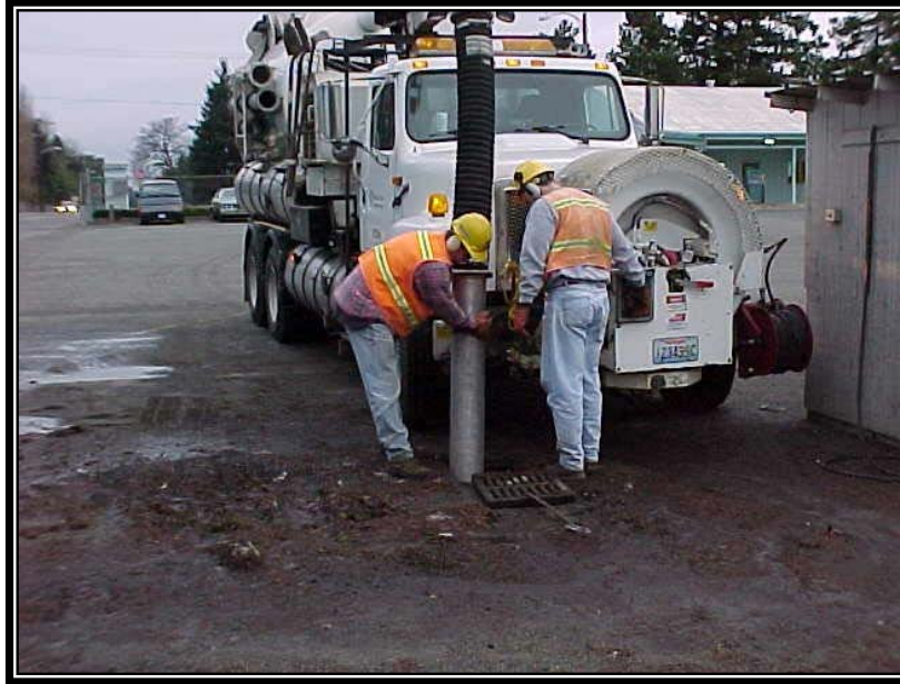
Figure 5.8. Catch Basin Cleaning with a Vacuum Truck.
