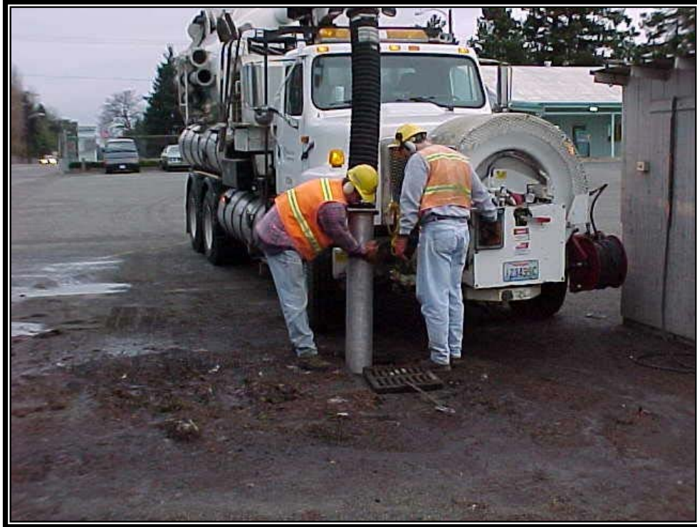
Figure 4.23. Catch Basin Cleaning with a Vacuum Truck.
