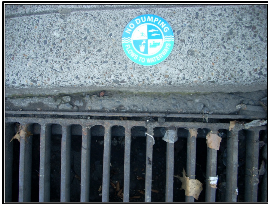
Figure 4.24. “No Dumping” Storm Drain Stencil.
