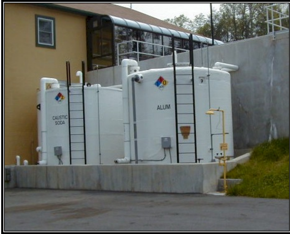
Figure 4.19. Aboveground Storage Tanks with Secondary Containment.
