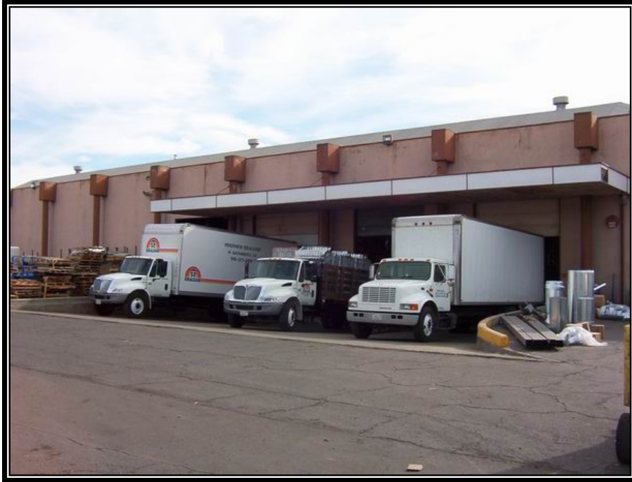
Figure 4.5. Loading Docks with an Overhang to Prevent Material Contact with Rainwater.
