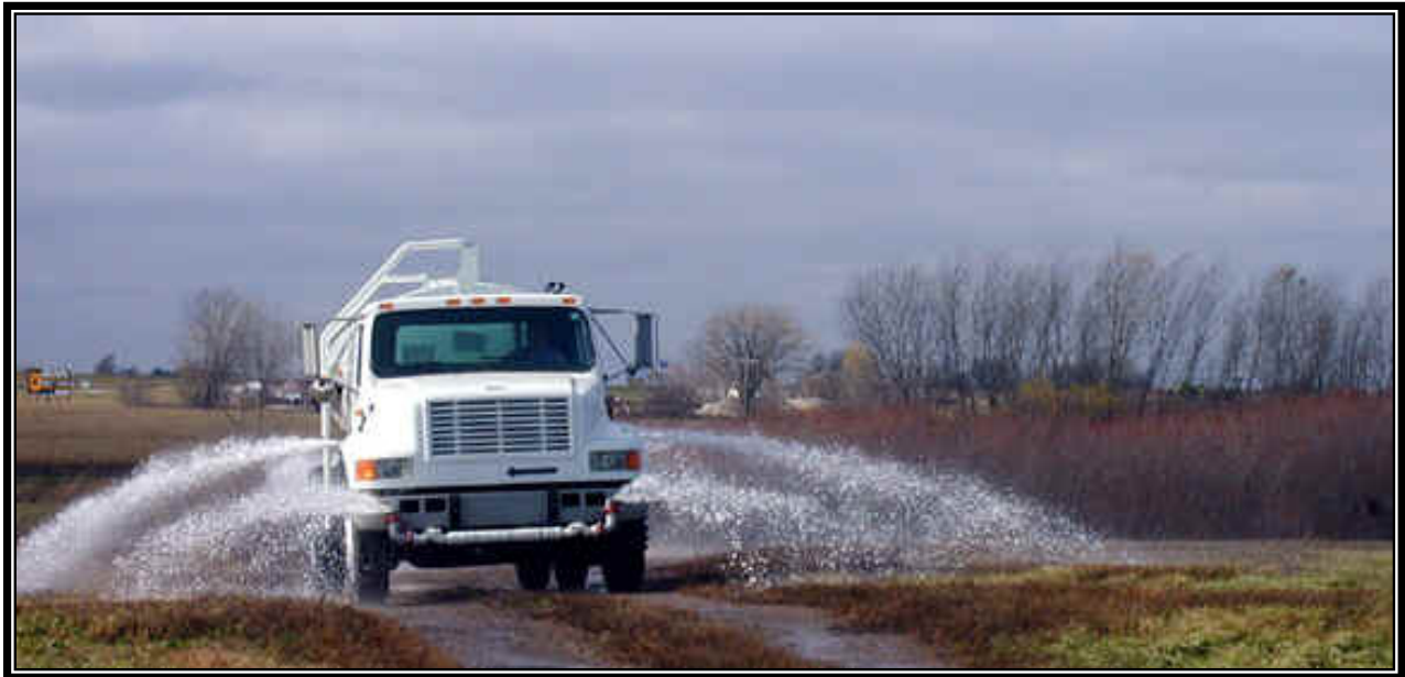
Figure 4.21. Dust Suppression by Water Spray.
