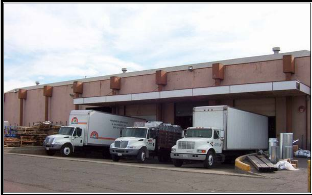
Figure 5.2. Loading Docks with an Overhang To Prevent Material Contact with Rainwater.
