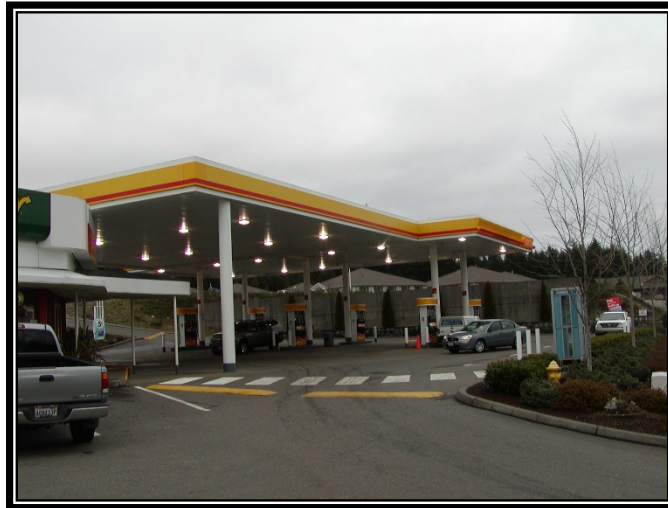
Figure 4.7. Roof at Fueling Island To Prevent Stormwater Run-On.
