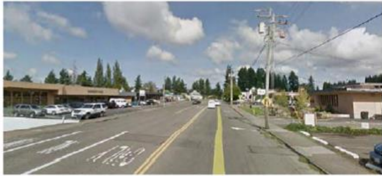
Figure 3.4: A road diet on Cleveland Avenue will include adding bicycle facilities, widening sidewalks, and installing street trees and stormwater facilities. The calmed streetscape allows easier pedestrian crossings and creates a more welcoming environment for mixed-use (re)development along the "main street".
